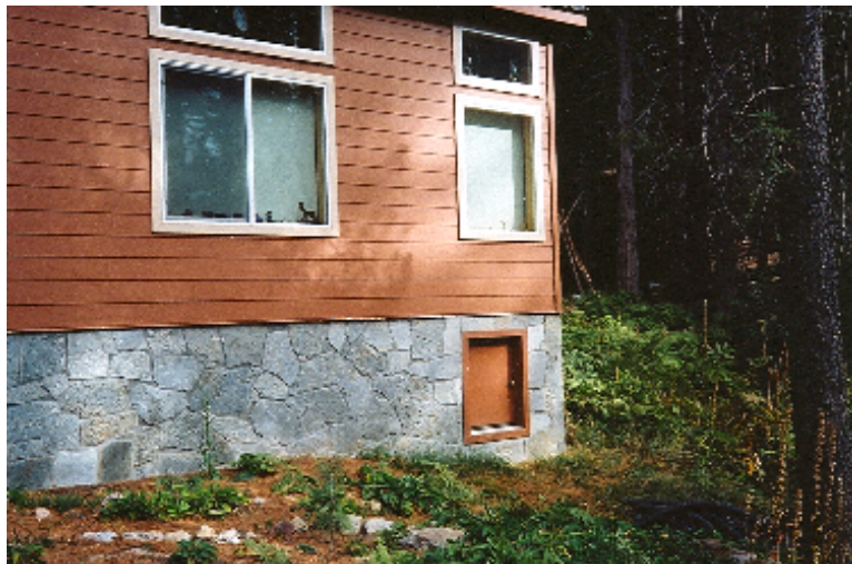
Perfectly Sealed Crawl Space on a Structure in Wilsonia Also Note the Fire Resistant Siding, a Cement Based Product
