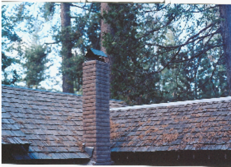
Pine Needles on a Shake Roof Make for a Flammable Combination
