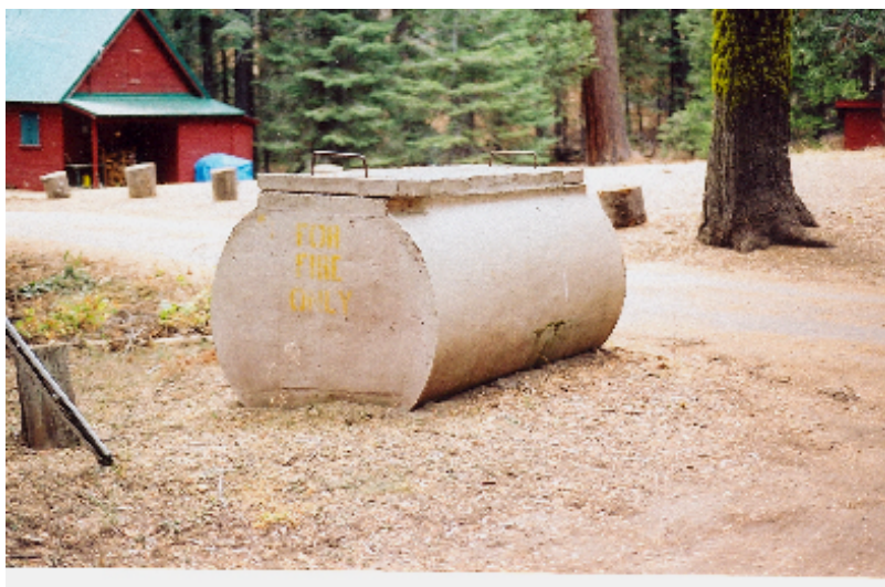
An Unserviceable 500-Gallon Water Tank
